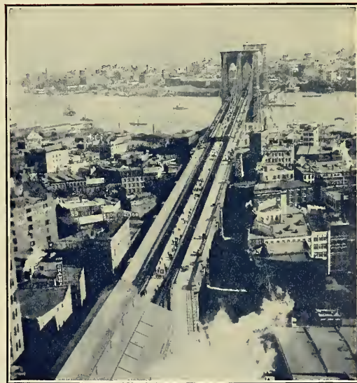
Brooklyn Bridge, New York Side
